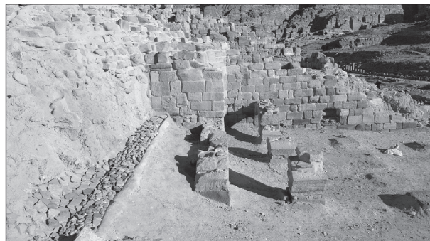
9. Southwest quadrant, showing covered drainage channel completed in December 2018 and areas of conserved walls, facing east (photo: Jack Green).
